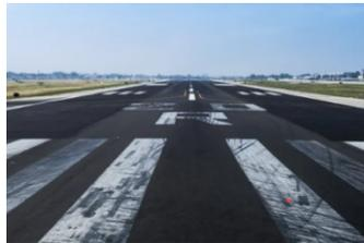
The activity required by our snowplow team to keep the runway and other airside access points clear during the winter, along with wear-and-tear from aircraft activity, takes its toll on the painted surface markings used to guide airplanes during take-offs and landings.
